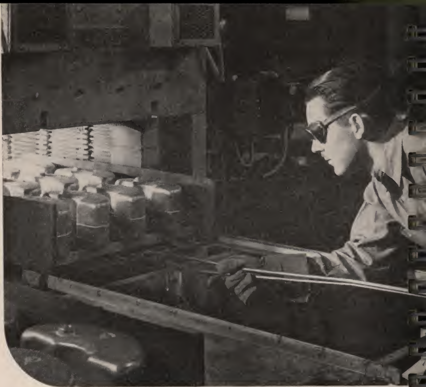
Furnace brazing gasoline tanks for outboard motors.
